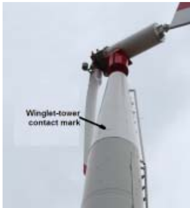
Fig. 2. Pictures of wind turbine after the incident a) lateral view; b) front view ; c) zoom on the impact zone
