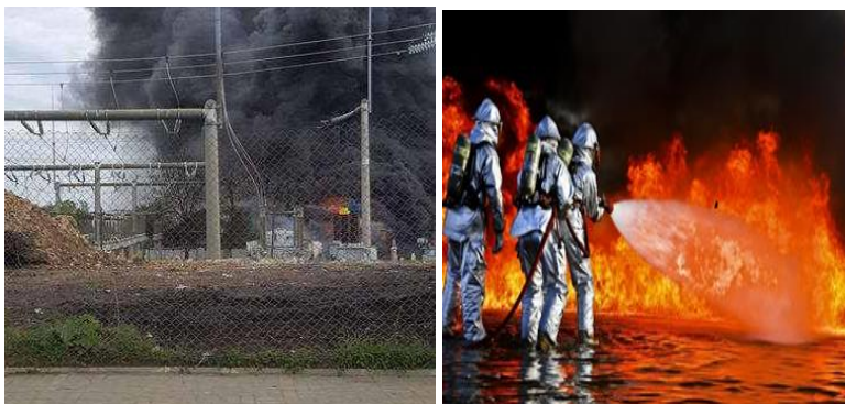
Fig. 1. Explosion and simultaneous fire of three power transformers in Botoșani city, RO [13, 14] - soil / surface water pollution by drain about 10 tons of mineral oil and air pollution by burning about 11 tons of oil
