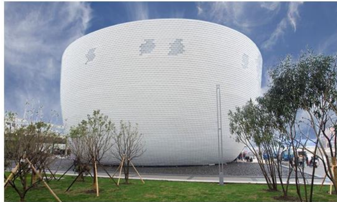
Figure 2. Application of WPC material (UPM ProFi) for shingle cladding (World Expo 2010, Shanghai) [2]
